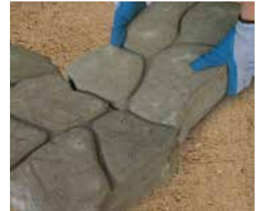
Step 4: Lay Patio Stones
